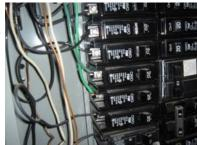
ESTIMATED COST \$75.00-125.00 Have a licensed electrician correct the use of a "green" wire connected to a circuit breaker. If any rewiring outside of the panel is required an added cost will be incurred.
