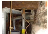
ESTIMATED COST \$150.00-250.00 each Replace the multiple temporary post jack at location. The use of a permanent post jack or 6 x 6 beam mechanically secured to the joist and floor are recommended. If a footing is necessary, as required, an additional cost will be incurred.
