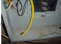
Correct the open splice in the middle of the basement and elsewhere as needed.
