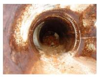
When a hot air furnace fails, has a defect in the heat exchanger or there is a defect or failure in the chimney system, the vent pipes to the chimney and the actual chimney, the distribution of deadly carbon monoxide gases may occur. You can't see or smell carbon monoxide, but at high levels it can kill in minutes". "Carbon monoxide is produced whenever any fuel such as gas, oil, kerosene, wood or charcoal is burned.
