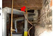
ESTIMATED COST \$50.00-75.00 Properly secure the vent from the water heater to the chimney. All vents should be mechanically secured at all joints and installed with an upward pitch of 1/4" per foot to the chimney. All vent piping must be of an approved material for the type fuel being used.
