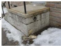
Some deterioration of the base to the side steps was noted and will require repairs in the next 1-2 years. As previously noted when the stucco is replaced these too should be repaired.
