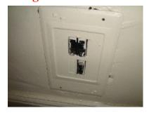
There are missing circuit breaker blanks in the electrical panels in various units. All openings must be properly sealed.
