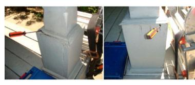
It was observed that the front right masonry pier was tilted more then is acceptable. While it is possible that this has been like this for many years, replacement is necessary with a proper footing. This must be installed by a licensed and qualified contractor.
