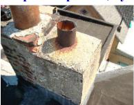
There are multiple abandoned chimneys present on the roof These should be sealed and stabilized. Failure to make these repairs will lead to water infiltration and result in possible additional damage.
