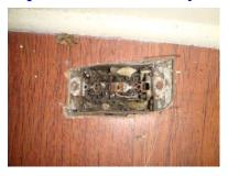
Correct and/or replace as maybe necessary the loose switch(s) in the bedroom of unit 7.
