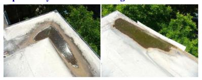
There is a large fixed skylight present on the roof. This unit has been covered with roofing material. When this is done, the body of the skylight can not be inspected. It should be assumed that ongoing repairs have been performed to the area in the past. Additional repairs and maintenance will be necessary in the future.
