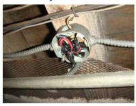
Correct the open splice above the suspended ceilings in unit 2.
