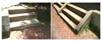
Railings are necessary for safety when there are (3) three or more risers. This condition exist for the front steps
