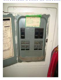
The sub panels throughout the building are improperly installed as per today's standards. All sub panels must consist of four (4) wires and have the neutral and ground isolated. In a normal panel the neutral and ground are both connected to the same point of termination.
