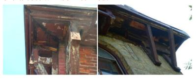
Along the lower roof edge of one of the roof it was noted that the wood was rotted and damaged and in need of replacement at this time. This beam is the support under the roof edge.
