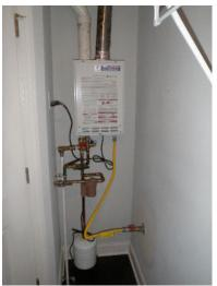
The intake and discharge pipes for the tankless water heater were poorly installed. The PVC intake vent pipe is cracked and broken inside and the stainless steel vent pipe was covered in what appears to be roofing cement. This does not appear to be a professional installation and must be corrected by a licensed and gualified contractor.
