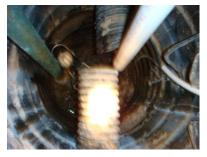
The sump pump discharges into the sanitary system. This is not permitted in most areas because this method of discharge poses an additional cost and burden on the sanitary system, all discharges should be to the outside placed a minimum of 3' and down grade from the building.
