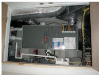
The heater is controlled in part by electronic zone dampers. This type system, when properly installed enables the control of the system from various thermostats by use of dampers and in some instances multi speed fans. The inspection, beyond a basic visible inspection is beyond the scope of a home inspection. As with any electronically controlled system some maintenance is to be expected. We recommend yearly inspections and preventive maintenance of these systems.
