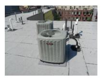
It was also noted that the pipes in which the air conditioner pipes and wires were fed through were poorly sealed and require repairs.
