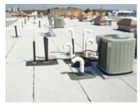
It was observed in the front of the roof and one of the neighbors roof that the capping had been patched, while all the other roof on the row were not. This is typically an indication of a past leak that may have been repaired. It is recommended that the builder be questioned as to reason for the patched area.
