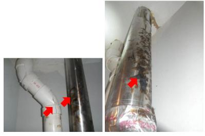
Inside the water heater it was observed that there is a small condensation leak present, This will in time rust the cabinet of the tankless water heater. This must be repaired accordingly.
