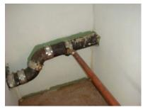
There are stains from what appears to be past water infiltration in the basement. At this time the there was no active infiltration, but this is not guarantee that under some condition they might not reoccur in the future. A determination of this type is beyond the scope of a visual inspection.
