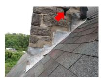
In some areas flashings were not visible. Typically a portion of the flashings are exposed above the shingles then installed to a wall. Without flashings leaks are likely. Since leaks were not visible inside, these areas should be monitored and if necessary installed.
