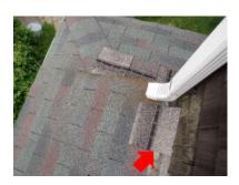
There are some shingles on the roof that are loose and in need of repairs at this time.
