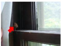
ESTIMATED COST \$100.00-125.00 each Repair or replace the failed window counter balance for the listed windows. When replacing the counter balances they should always be replaced as a set.
