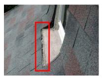
The trim in various areas show signs of deterioration and will require replacement. It is recommended after replacement that all area be covered with aluminum to reduce future maintenance.
