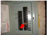
The sub panel, in the basement is improperly installed as per today standards. All sub panels must consist of four (4) wires and have the neutral and ground isolated. In a normal panel the neutral and ground are both connected to the same point of termination. Although there are four wires the neutral and grounds are not isolated.
