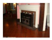
The fireplace in the second floor office appears to have been modified and should not be used until inspected and certified safe.
