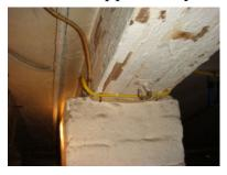
The sub flooring is tongue and grove flooring installed on a diagonal and was visible inspected for less then 5%± of the area. This is a superior method of installation and normally will produce a strong flooring system.
