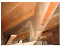
There are visible failed or compromised joist present that were *improperly repaired* in the past. The joist are located in the basement. Proper repairs are necessary at this time.
