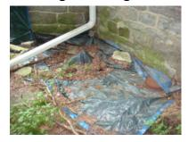
On the left side of the house there is a aluminum downspout that is loose and not properly supported. This must be repaired as necessary.
