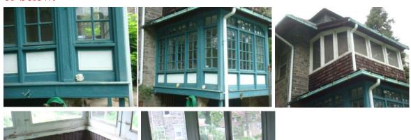
The wood insills for the accessible windows, in some areas, were in poor condition. Failure to properly maintain these areas will lead to failure and water infiltration. It is recommended that all sills be properly painted and repaired on an as needed basis. Some areas may require additional repairs prior to painting, the cost of repairs or replacement will be additional.
