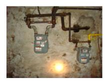
The limited visible piping is copper and shows no signs of excessive deterioration inconsistent with the age of the building.
